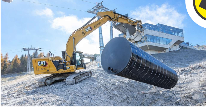
Retentionstank Regenwasser
