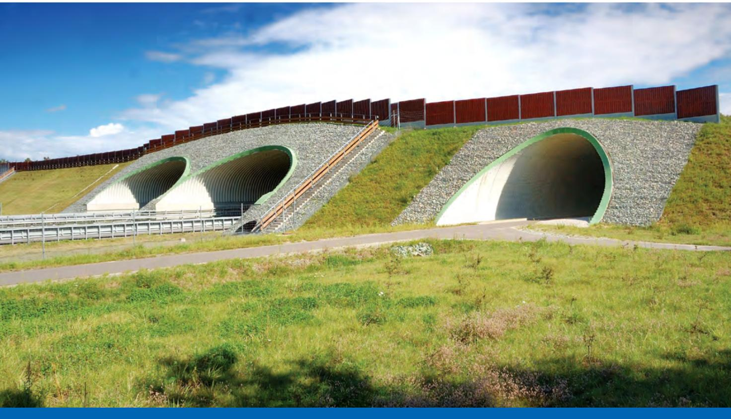
SuperCor® versatile structures are used for roads and railways and industrial applications as well as for reinforcement and reconstruction of existing structures such as:
