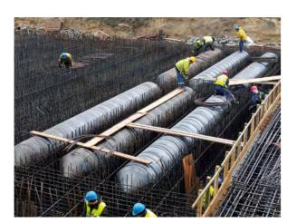
Coating steel with a polymer film, called Trenchcoat™, Trenchcoat™ film can be applied on either one or both sides
